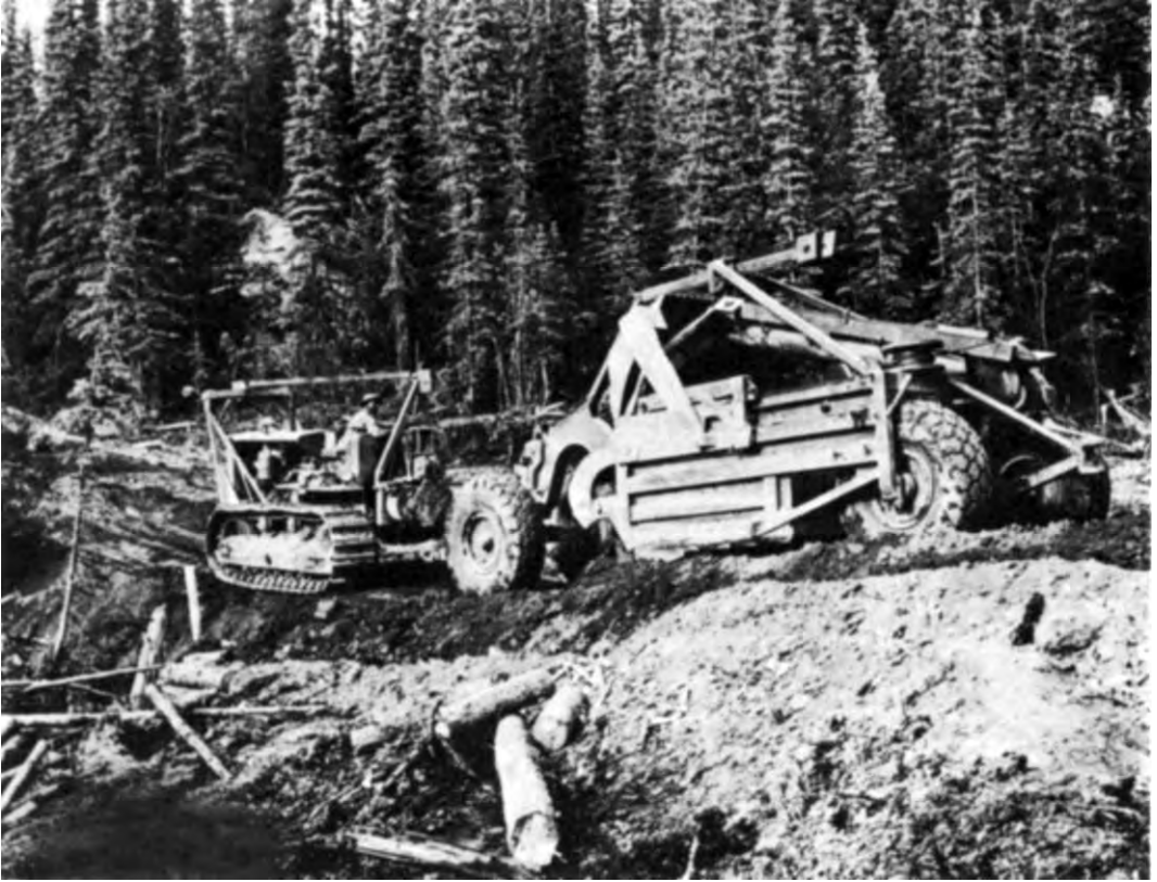
OPERATING HEAVY EQUIPMENT ON THE ALASKA HIGHWAY
